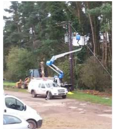
Western Power upgrading the electricity
